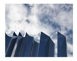
ALUCOBOND (OR SIM) RAINSCREEN PANELS WITH MIRRORED ALUMINUM FINISH
