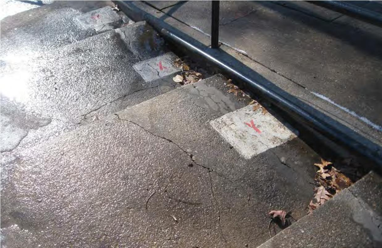
Characteristic settlement cracking East Loge seating base.
