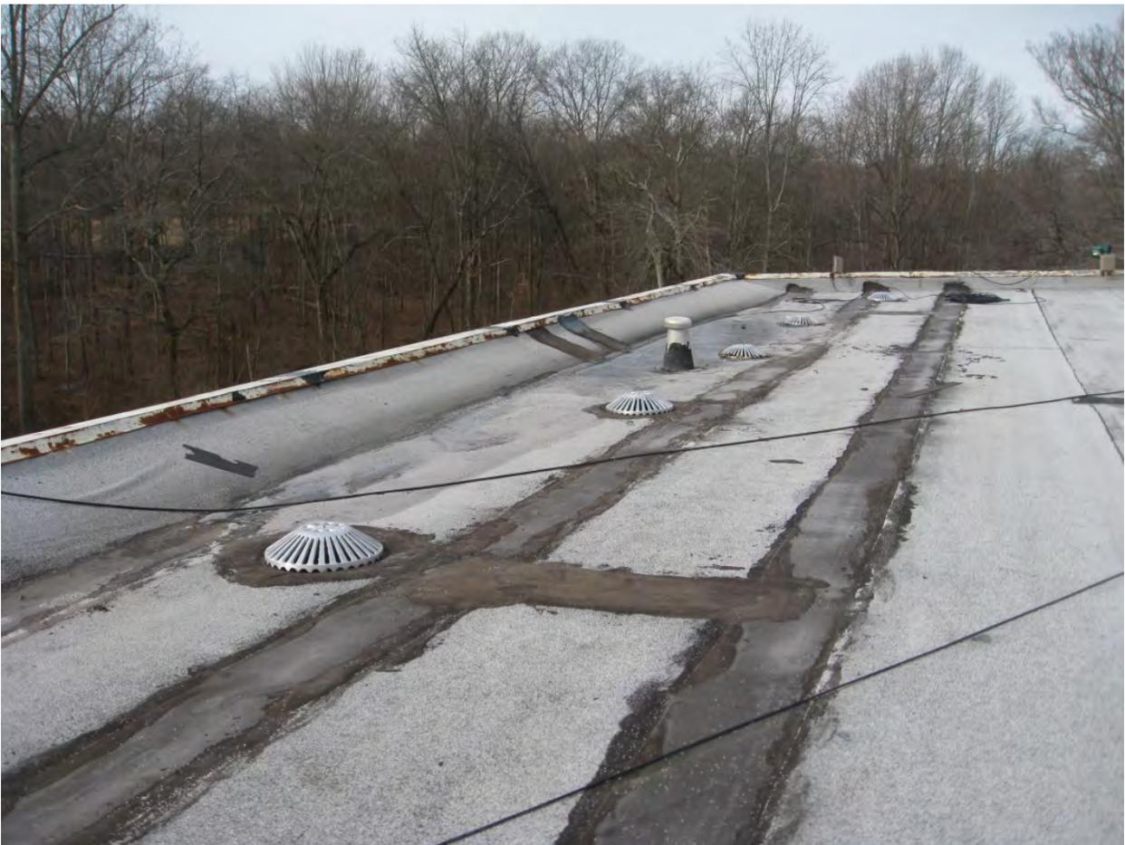
View of Pavilion roof above rear of stage. Roof, flashings and drains are now in need of replacement.
