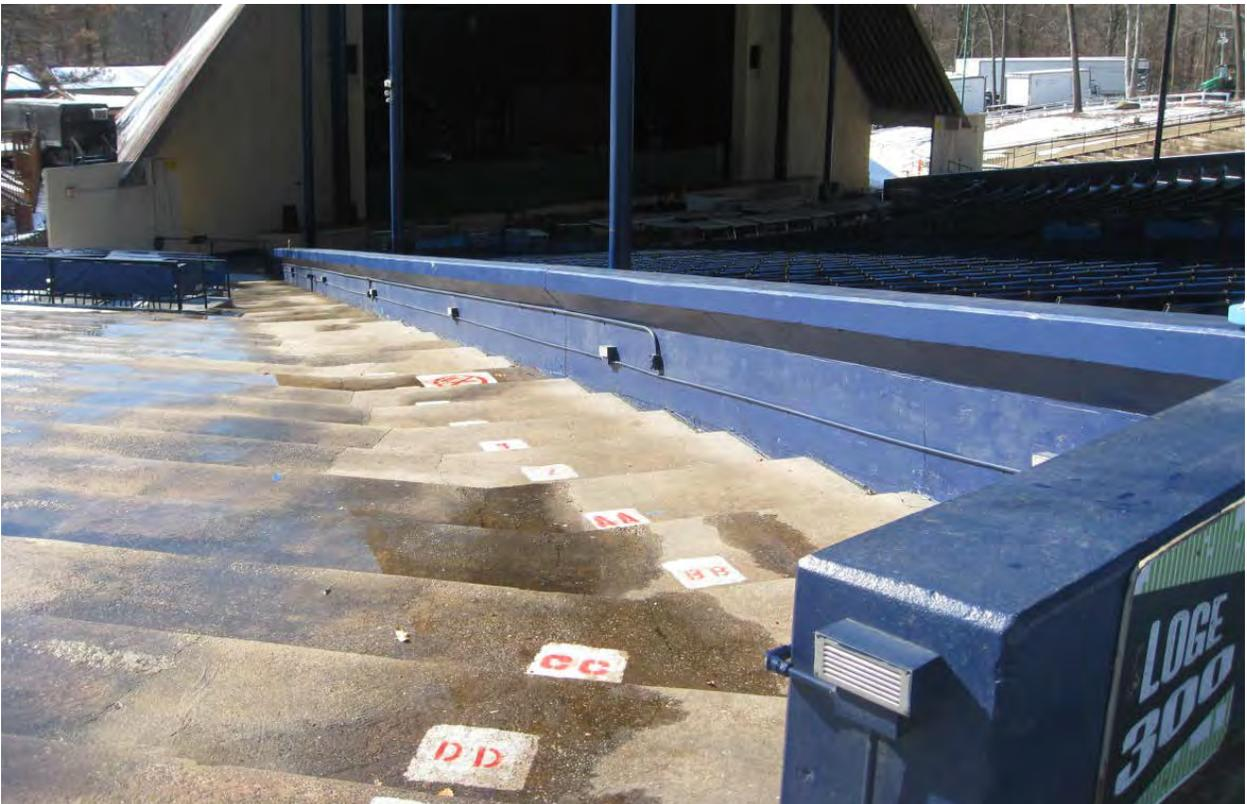
Original concrete cheek wall between original and newer Loge seating obstructs ingress/egress.
