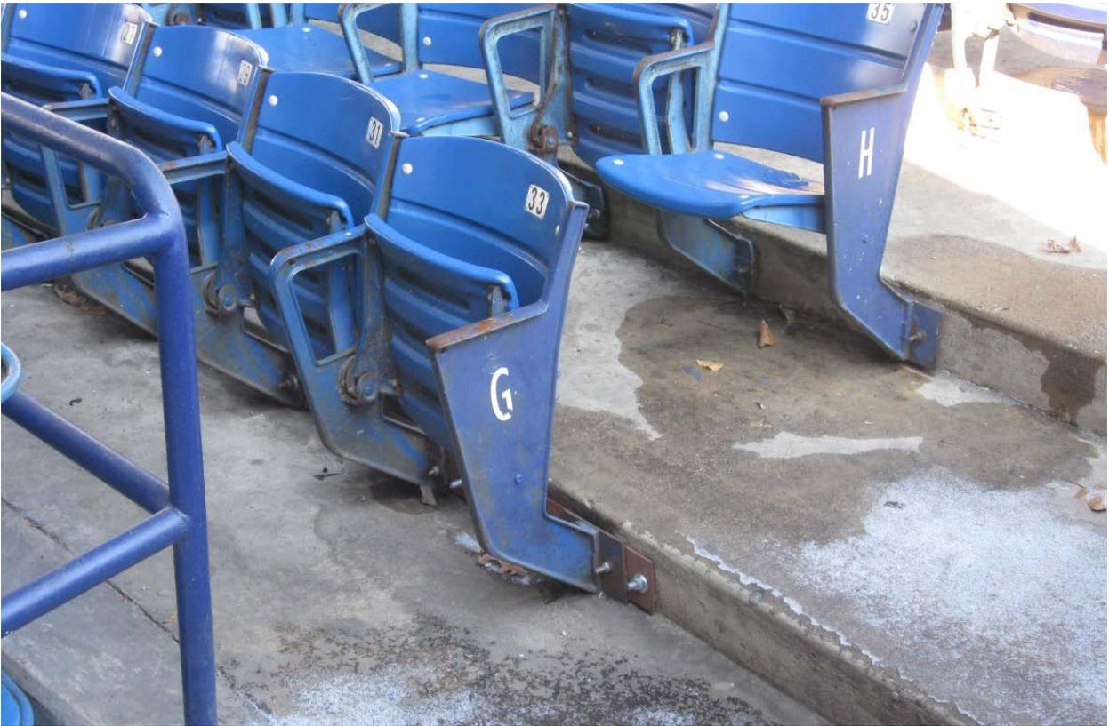
Replacement parts for original riser-mounted cast iron seating have run out.
